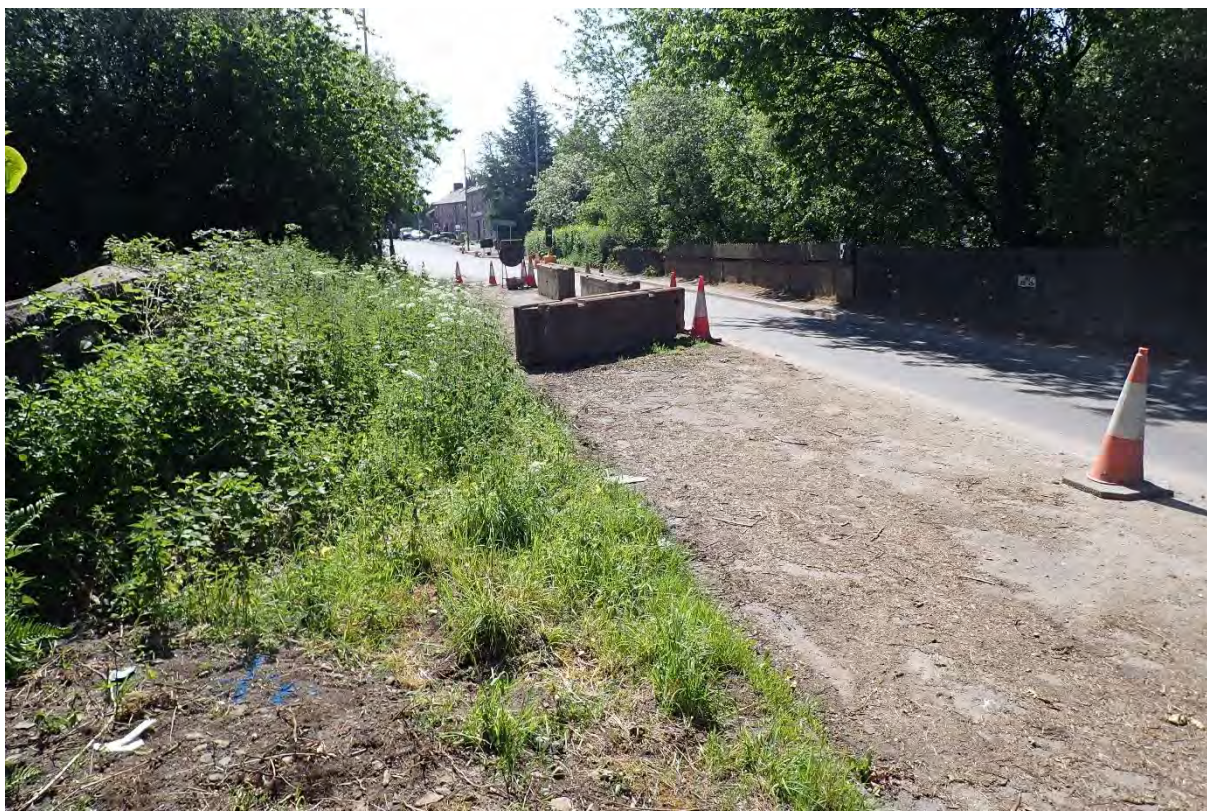
12. Photo looking south showing the carriageway surface and highway verge
