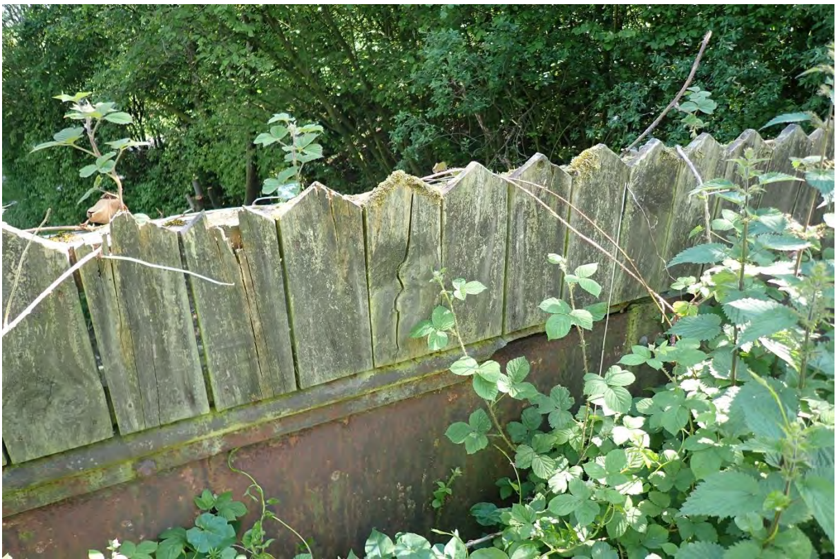
10. North East parapet
