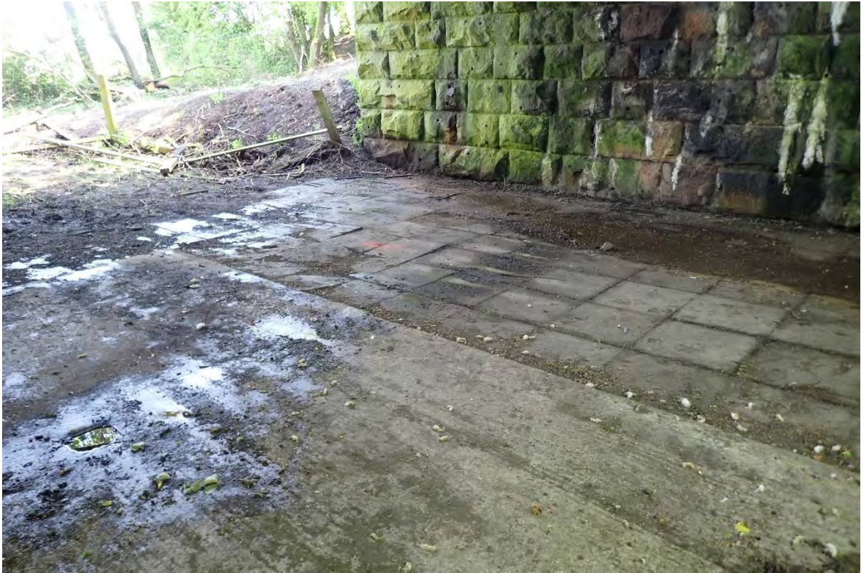
43. Surfacing under the bridge
