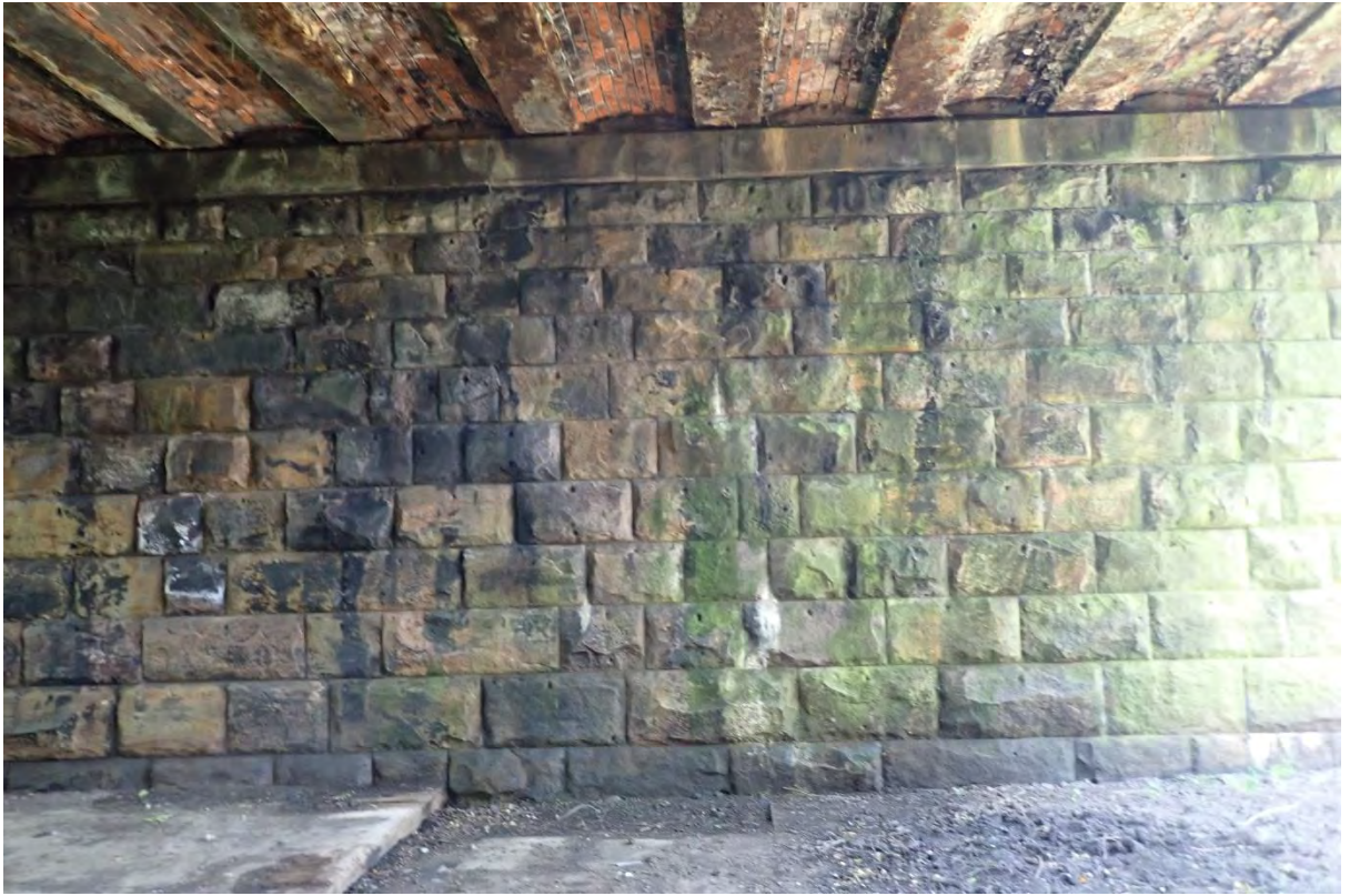
37. General view of the NW abutment
