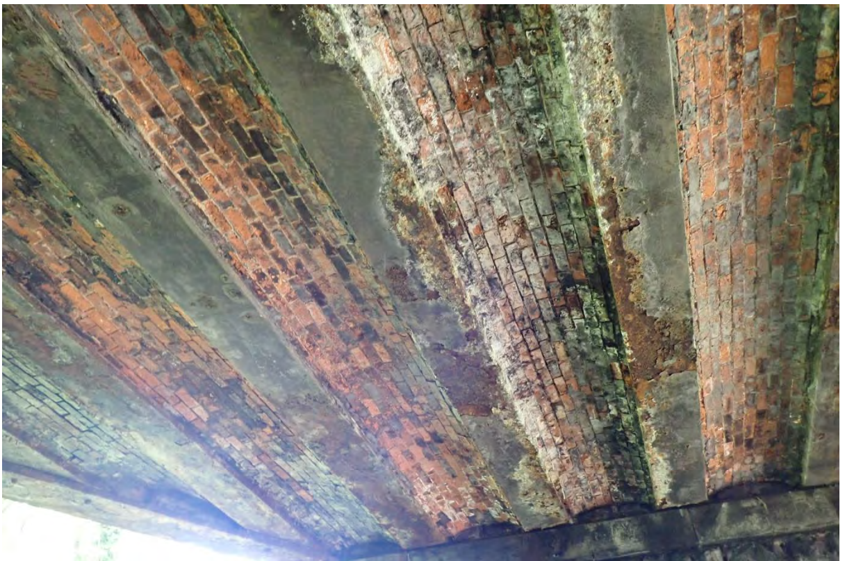
22. General view of the cast iron girders and brick back arches
