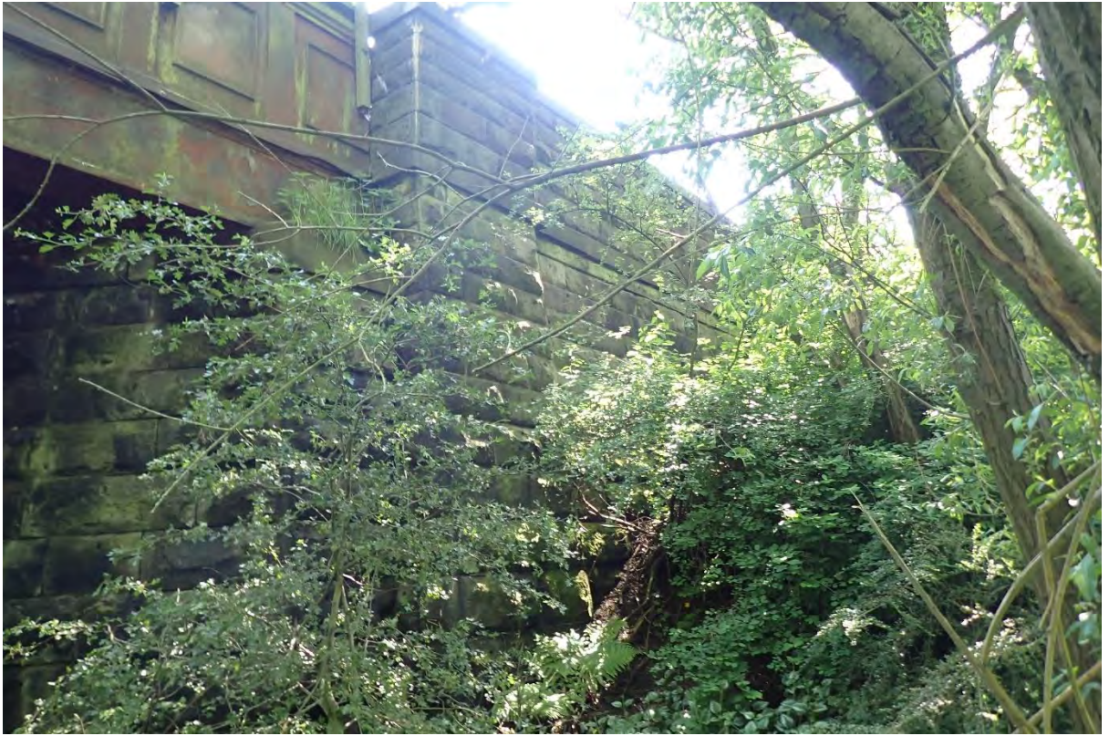
41. SW wing wall and embankment
