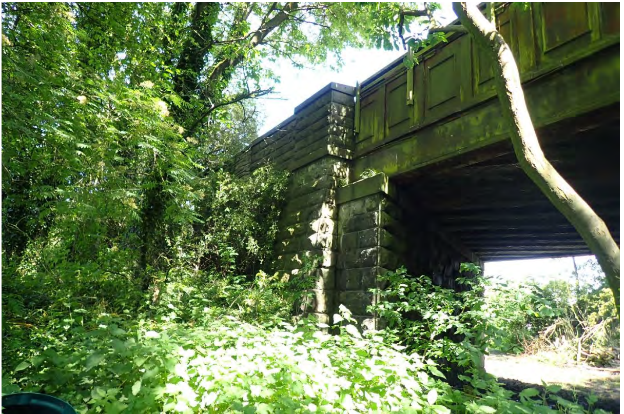
42. NW wing wall and embankment
