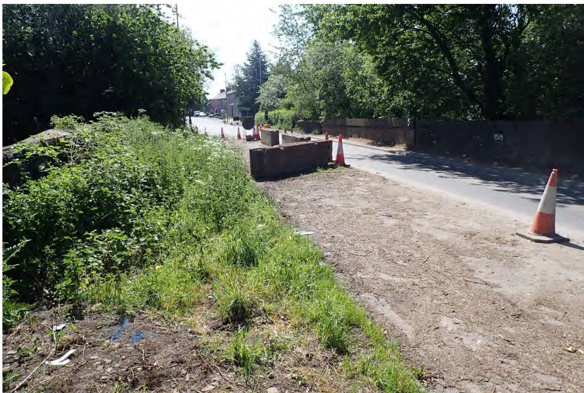
2. Photo over the bridge looking south along the A675
