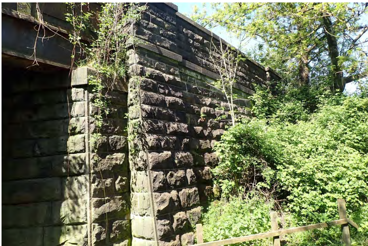
40. NE wing wall and embankment
