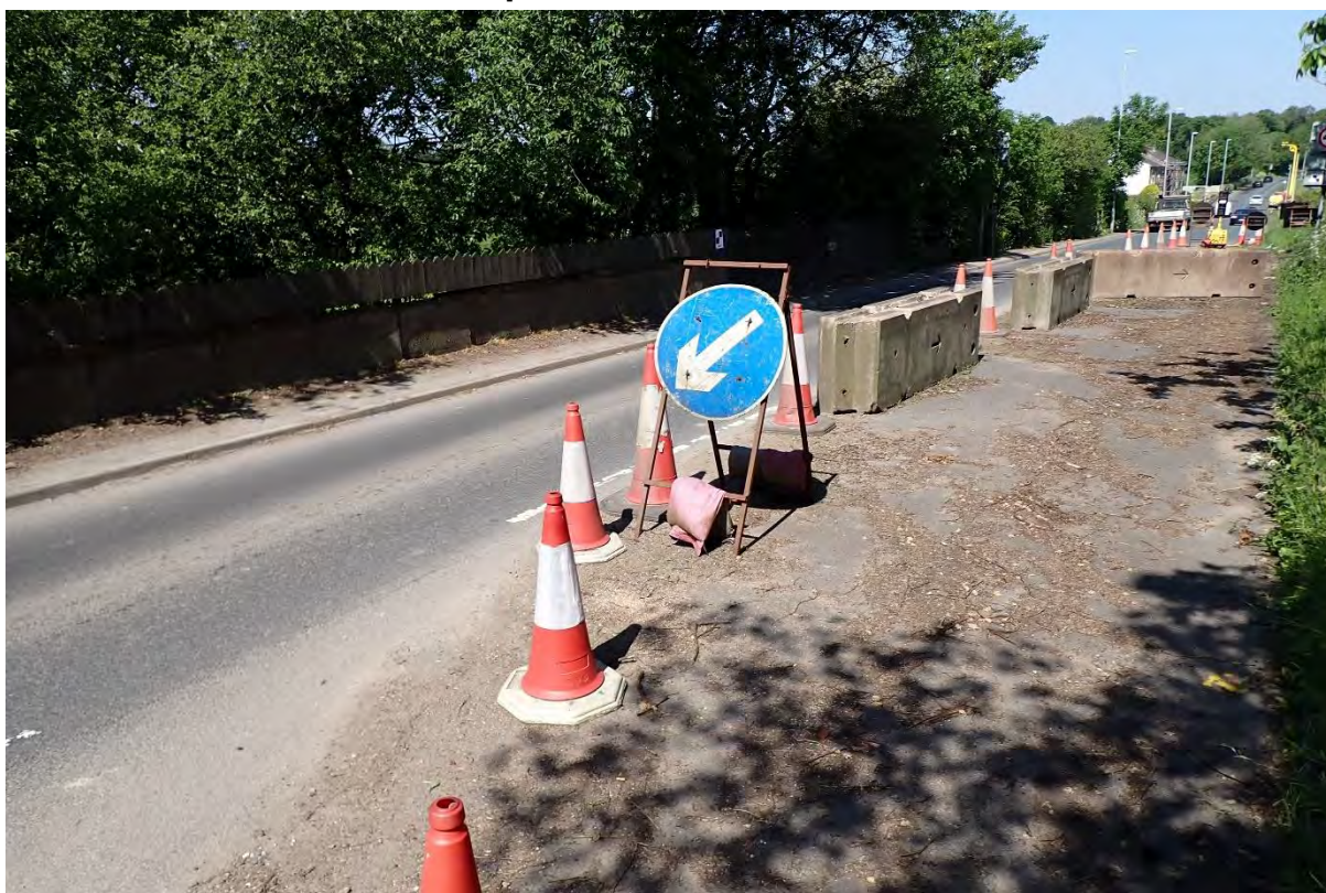
1. Photo over the bridge looking north along the A675
