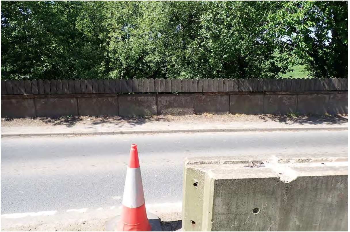
9. South West parapet
