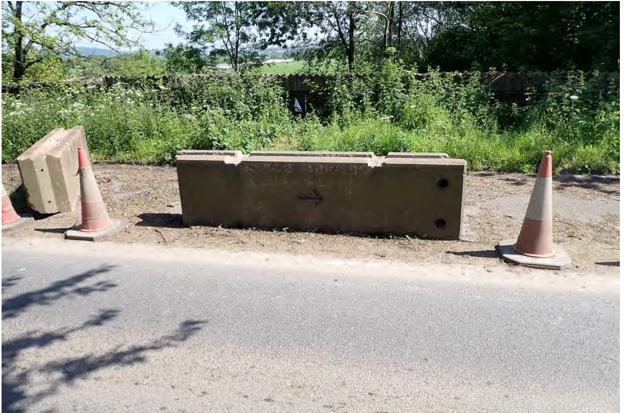
5. View of highway surface with temporary traffic measures in place
