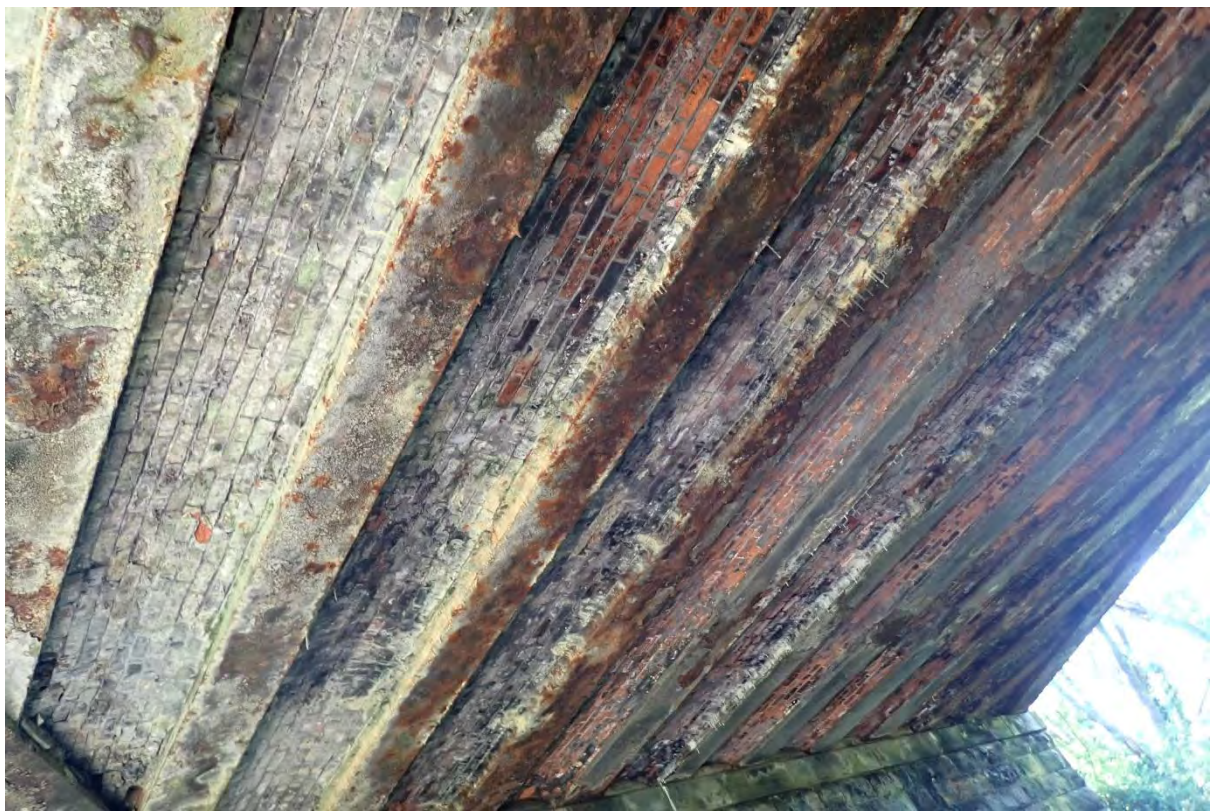
16. General view of the internal deck beams and brick jack arches
