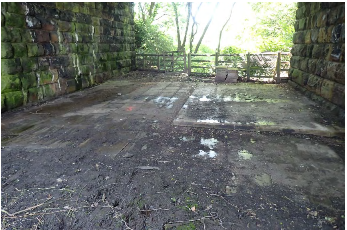
44. General view of the flagged and concrete surface under the bridge
