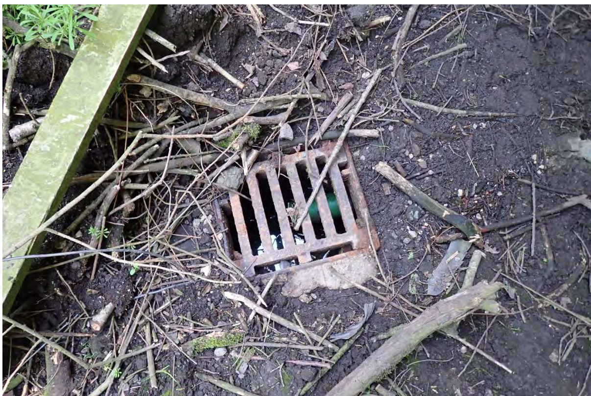
45. Drainage gully under the bridge is clear of blockages
