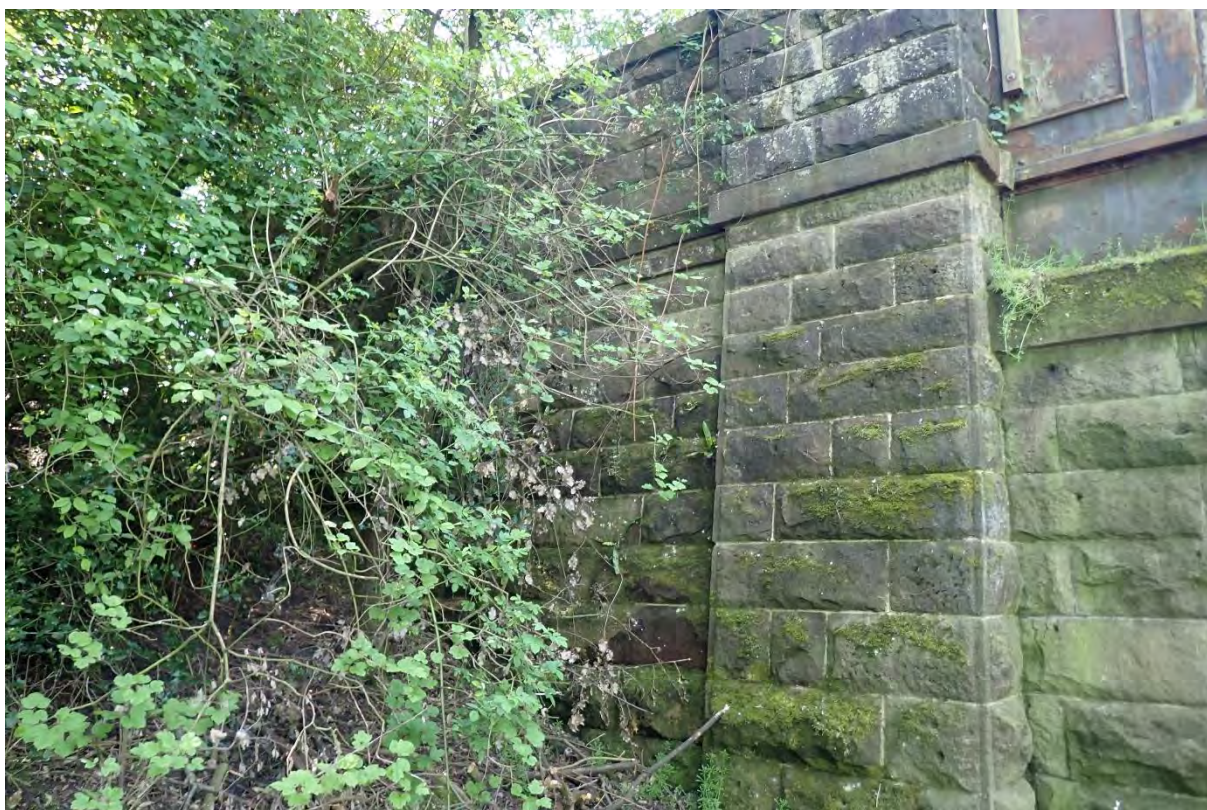
39. SE wing wall and embankment
