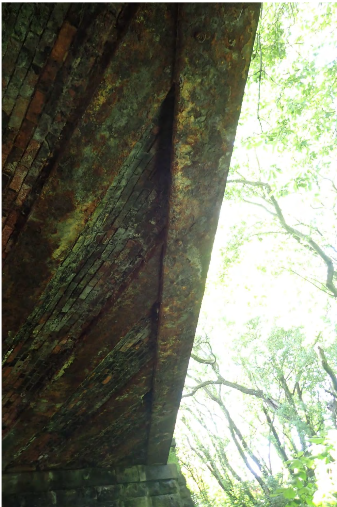
27. External end beam (west)
