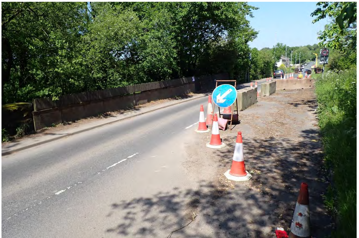
8. View over the bridge showing the highway surface and current temporary traffic restrictions
