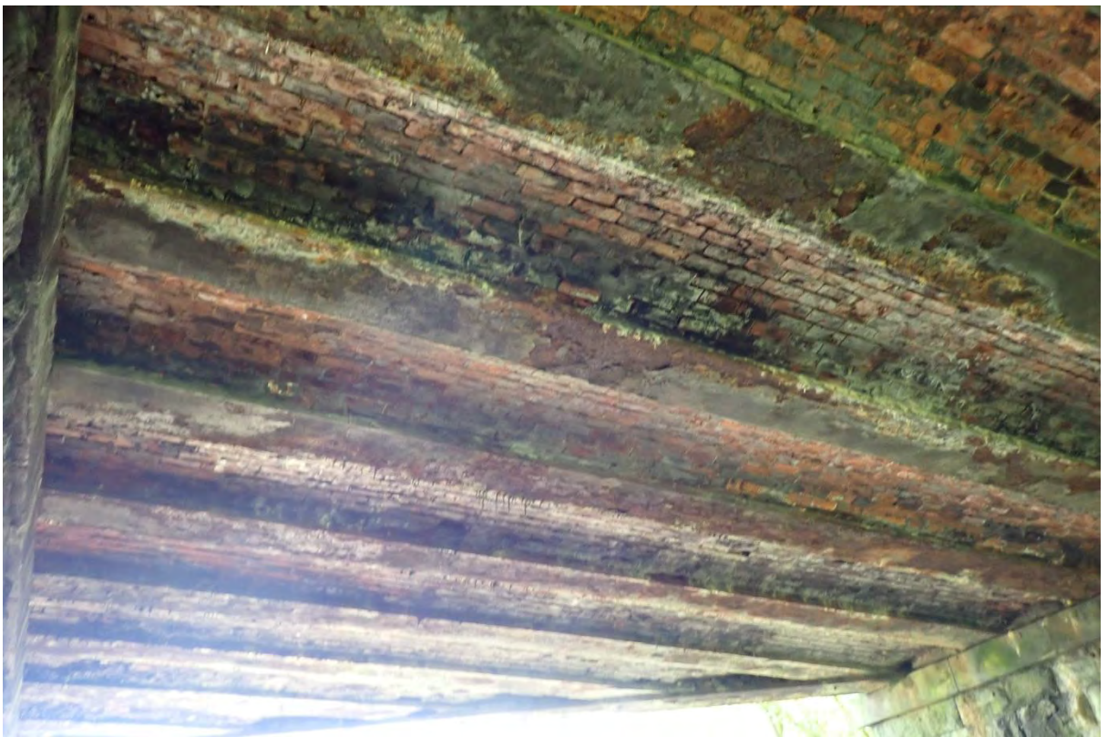
26. General view of the deck looking eastwards
