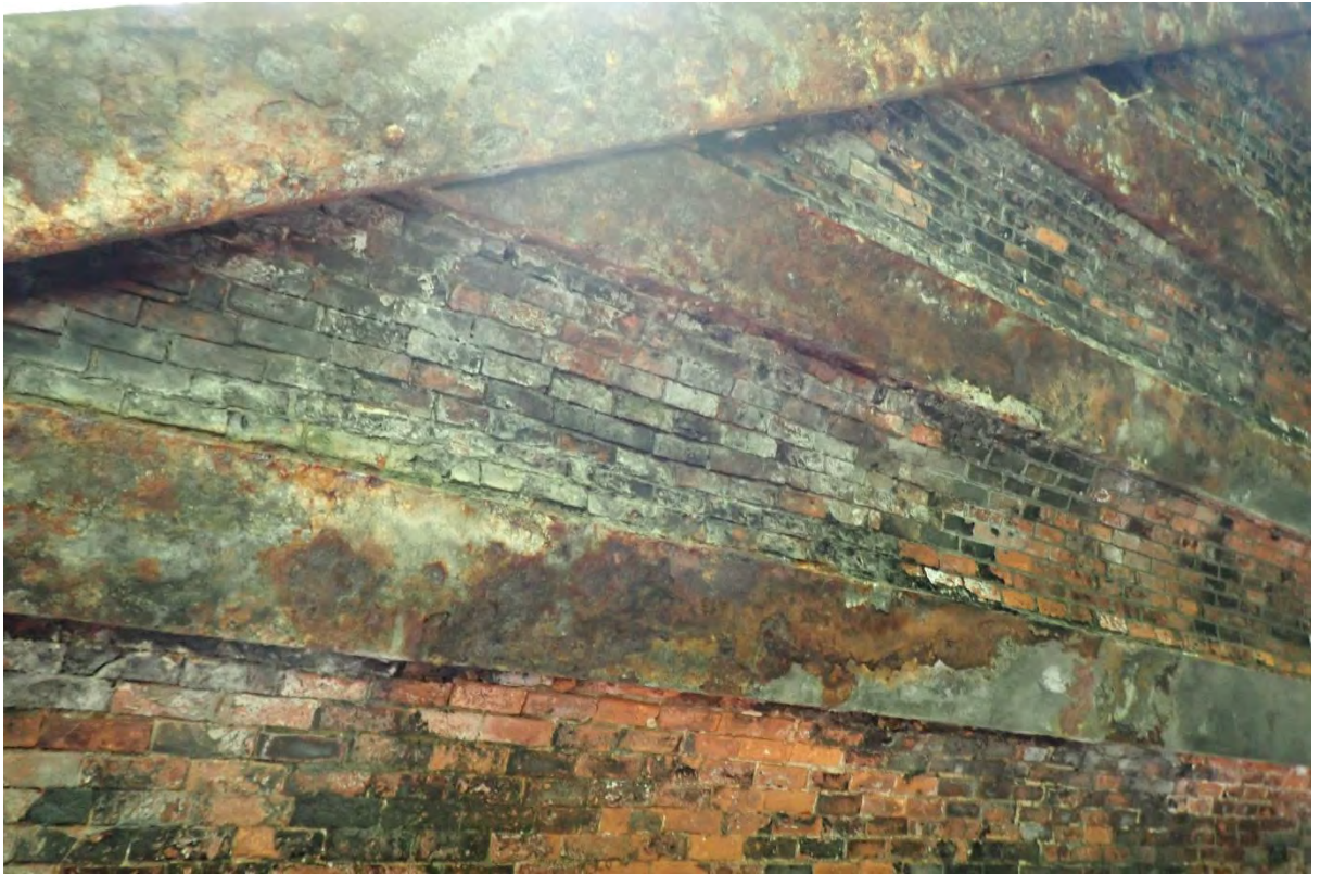
25. Overview of deck elements
