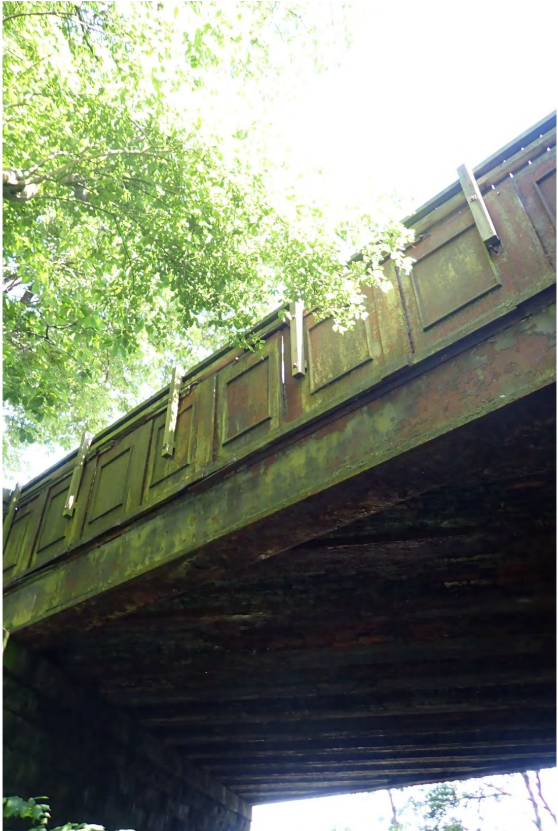
29. Overview of the west end of the bridge
