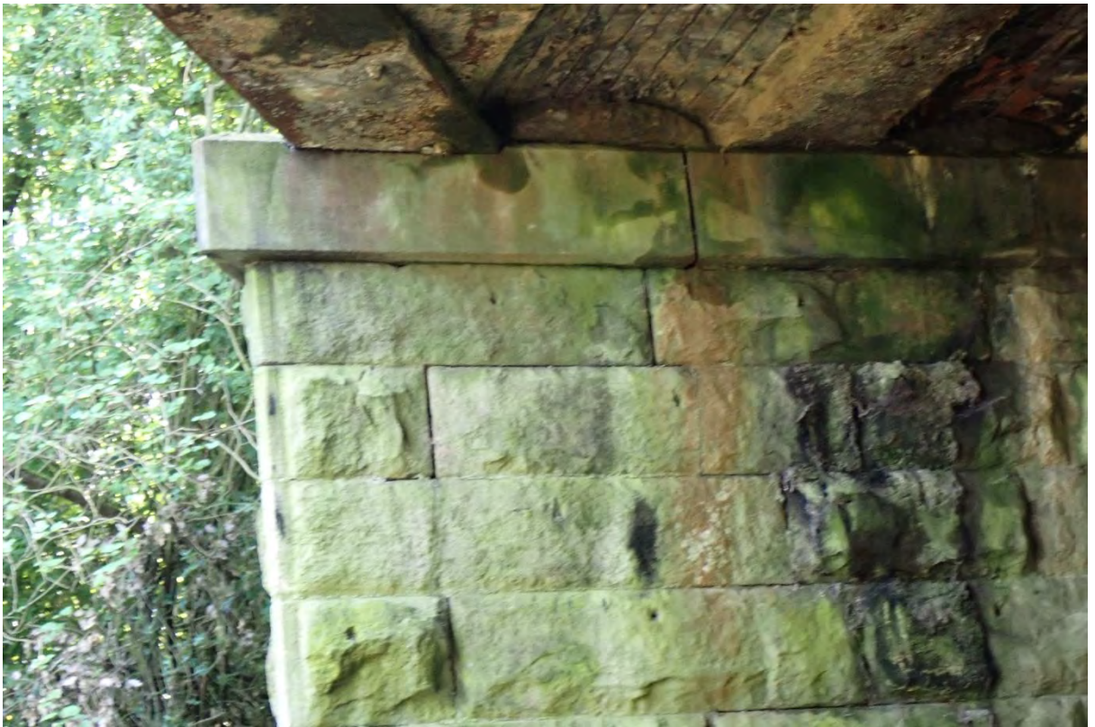
38. Photo of the SE abutment and stone bearing plinth
