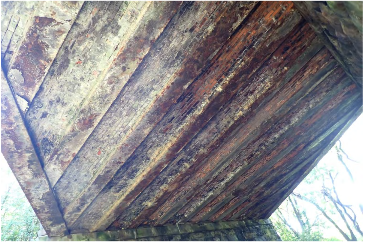
19. General view of the cast iron girders and brick back arches
