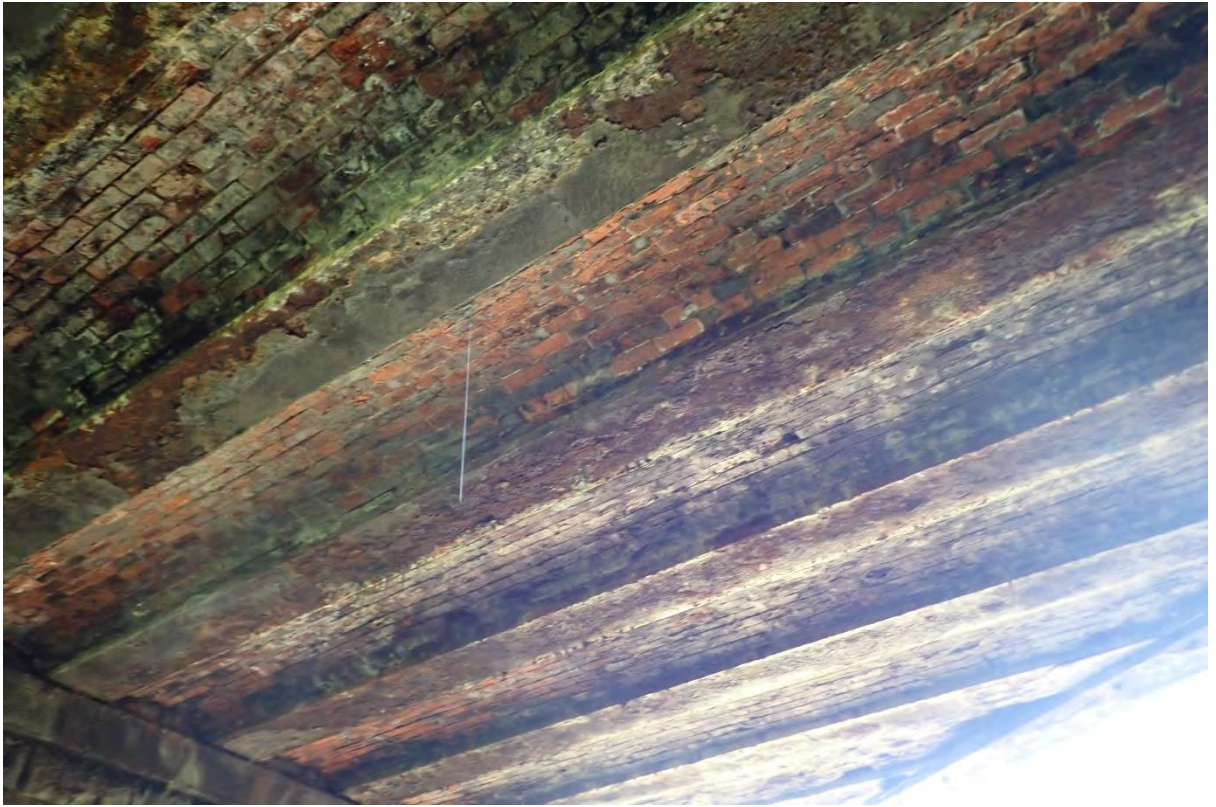
23. General photo of deck elements
