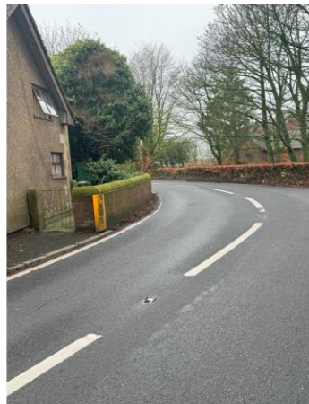
Fold House Corner A588 post repair Damage to newly added post
