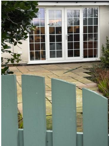
Proximity of Hillfield House main living Area to the gate to the road
