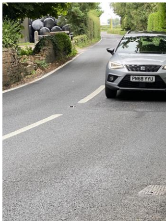
Fold House Corner A588 pre repair
