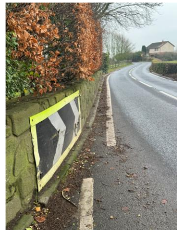
Fold House corner opposite the Post – damaged warning sign
