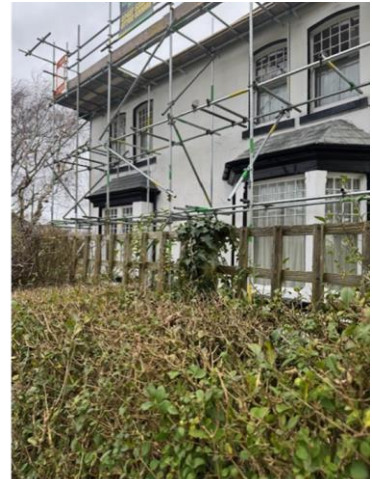
Proximity of Pointer House to the road
