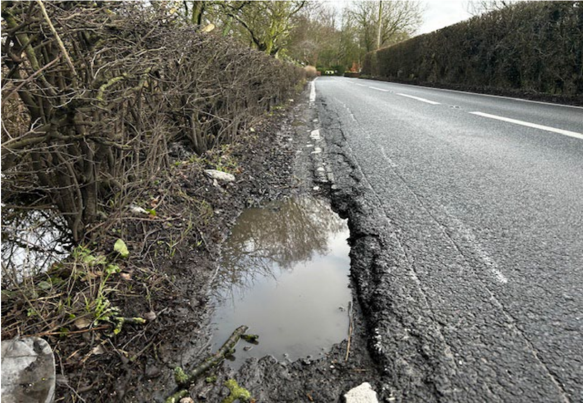
15- Adjacent to the access serving Heyswood House - Carriageway edge deterioration/ pooling
