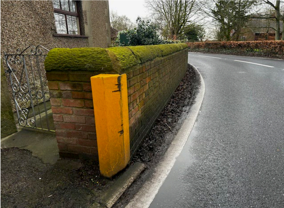
19- Adjacent to the Access serving Fold House – Damaged wall protector
