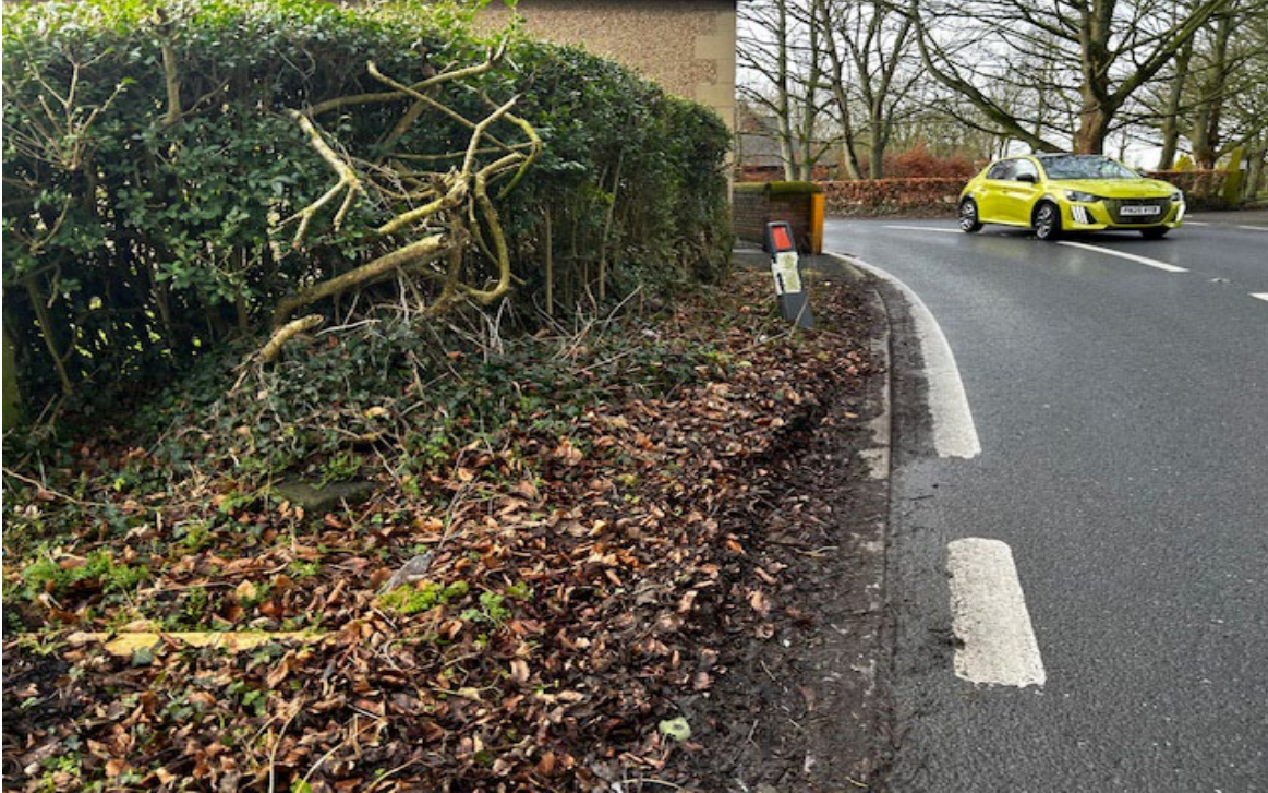
23- Opposite the access serving Fold House Farm- Verge overrun at bend in road/ damage to verge marker posts
