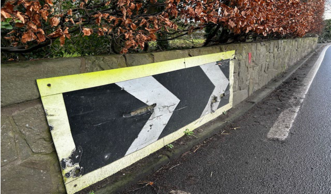
19- Adjacent to the Access serving Fold House – Damaged wall protector
