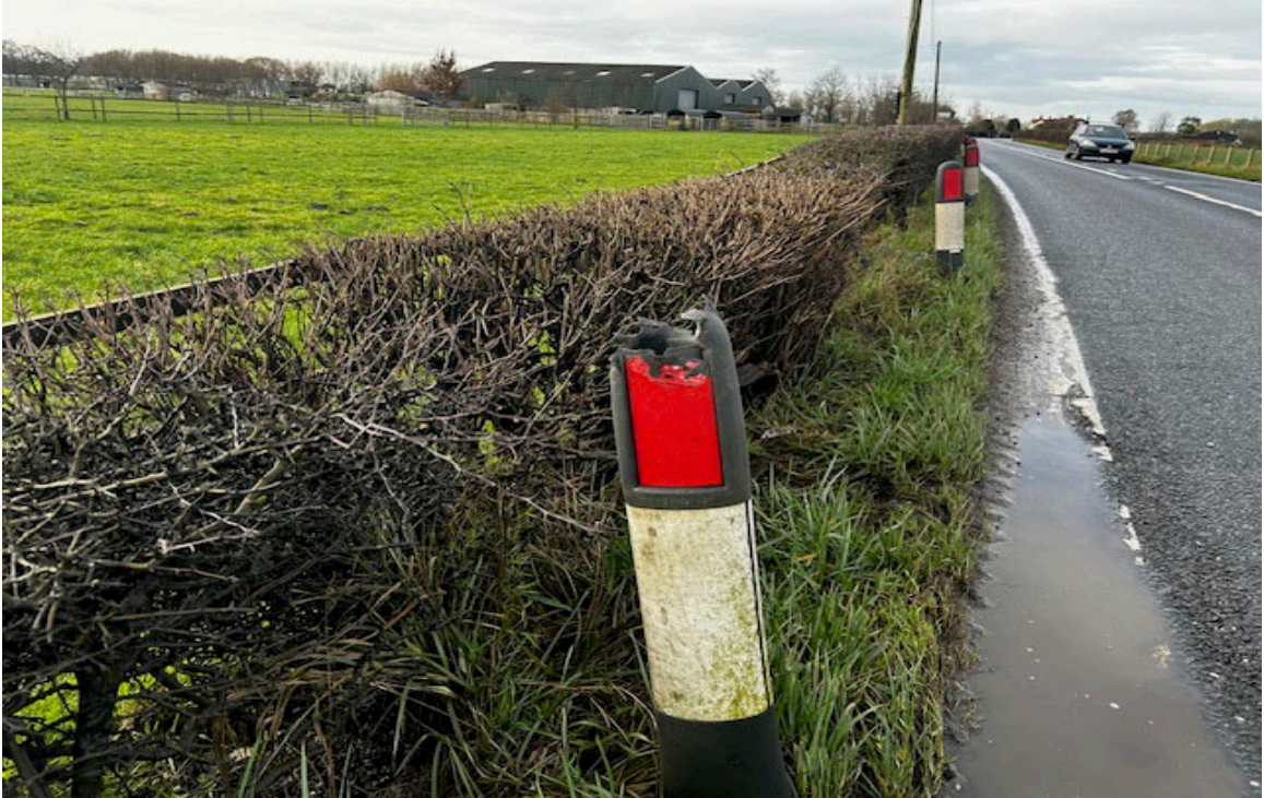
15- Adjacent to the access serving Heyswood House - Carriageway edge deterioration/ pooling
