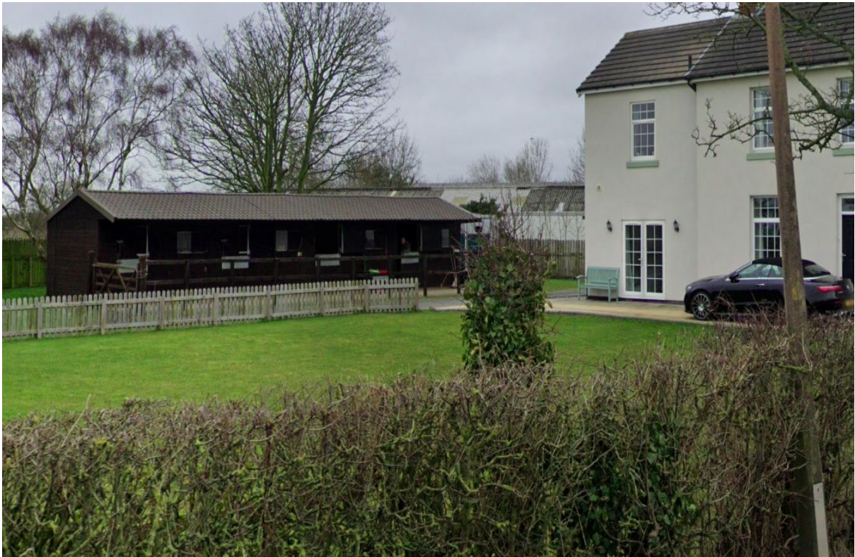
1 - Hillfield House, Lancaster Road - Stables
