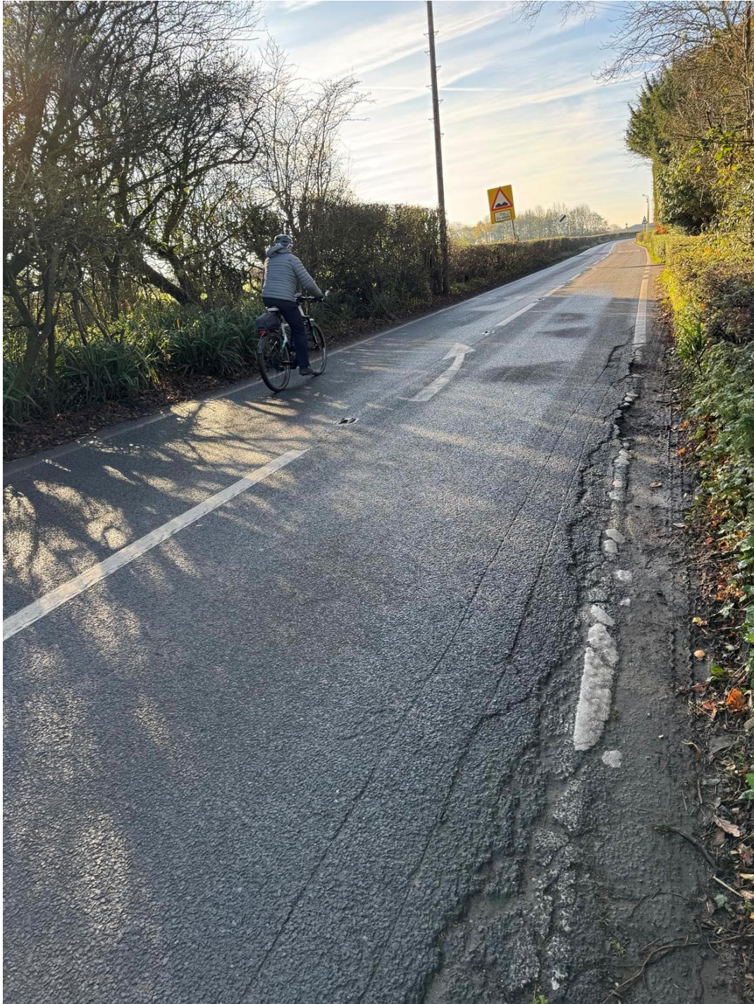
Photograph 1: Picture shows a cyclist using the network and verge overrun (Image from the site visit conducted on 14 th November 2024).
