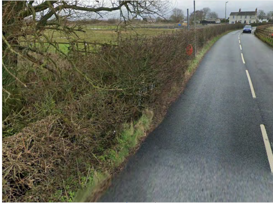
Bush Overgrowing onto Highway Cut Back In Line With Hedge Either Side. Tree Overgrowing Highway Trimmed to Highway Clearance Height
