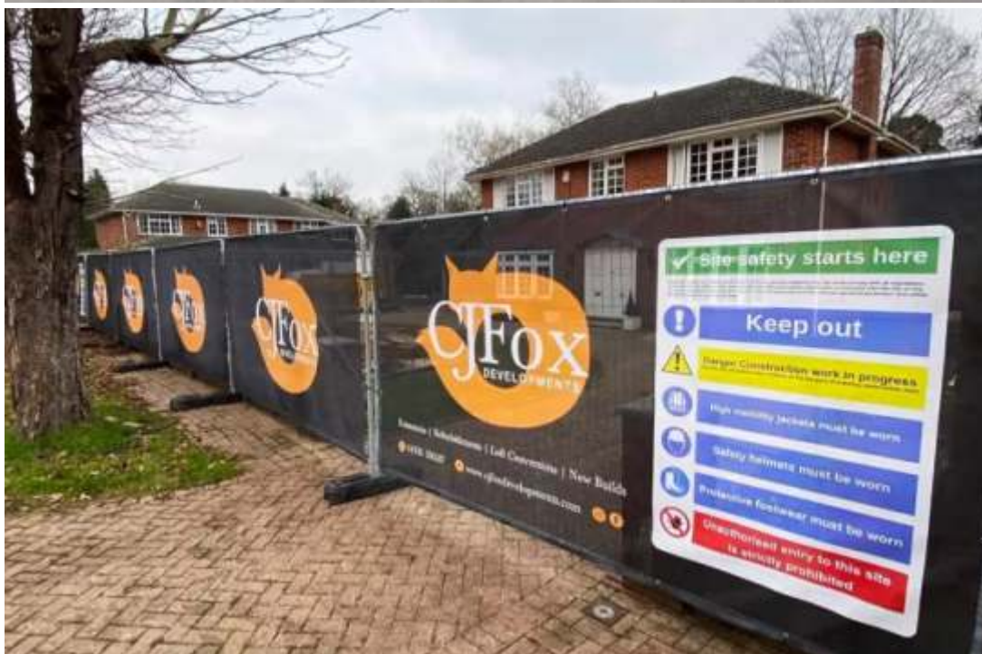
Plate 16 Examples of Heras Fencing with mesh screen
