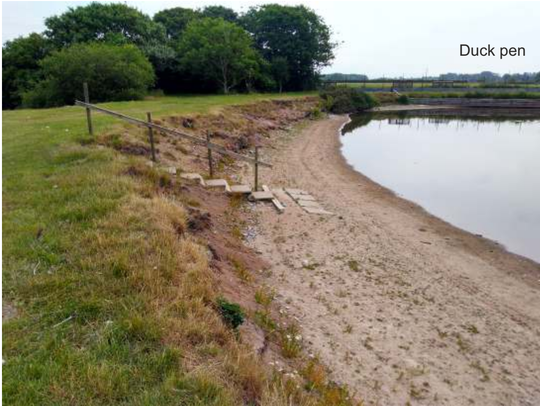
Plate 1 Summer - north bank looking east
