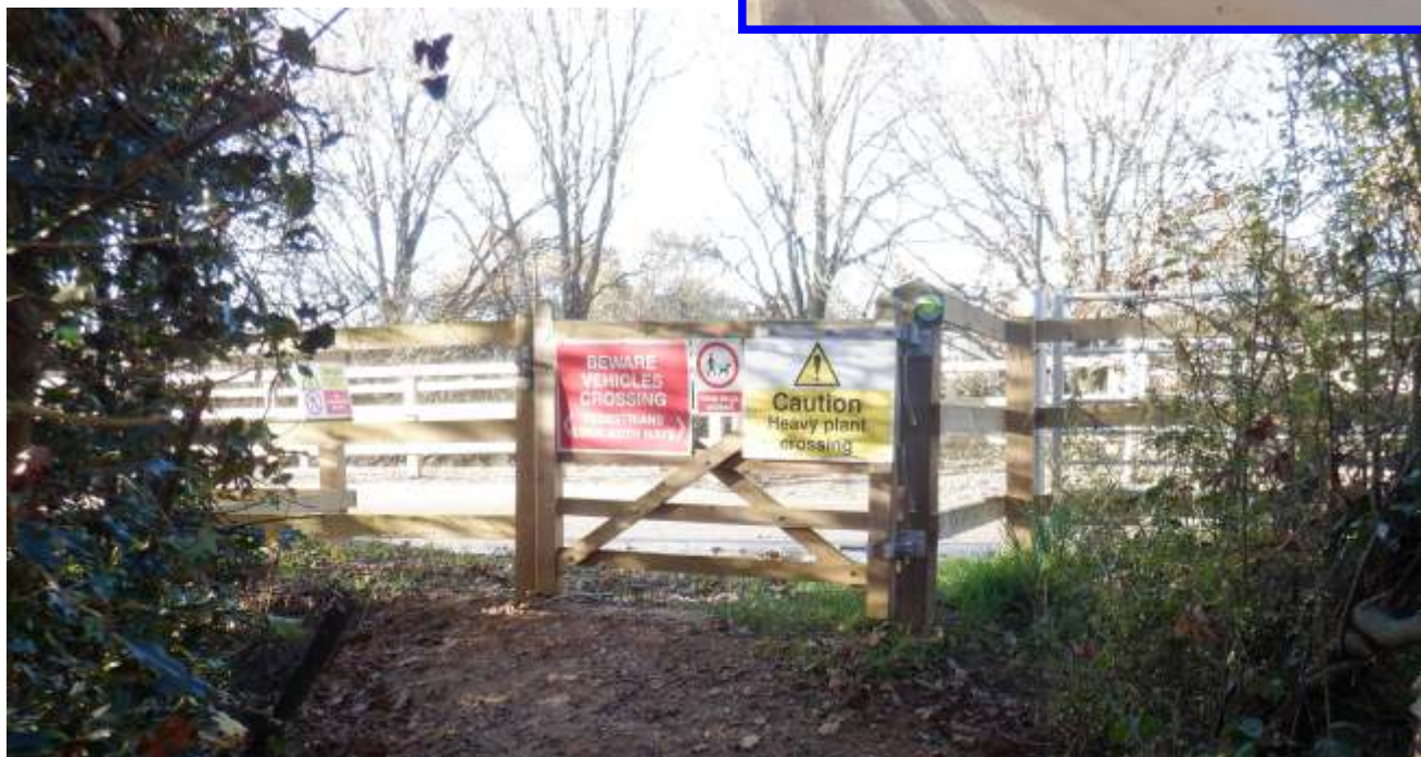
Plate 13 - Footpath crossing of new access road- signs & gate
