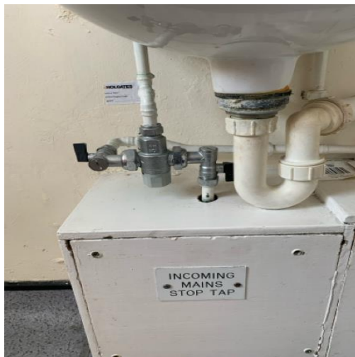
TMV 01 (Ground floor accessible WC)
