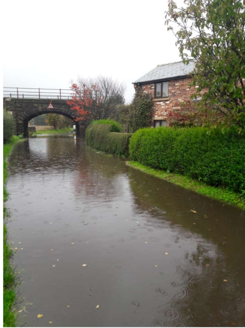
Figure 1: Warpers Moss Lane flooded under railway bridge, October 2020
