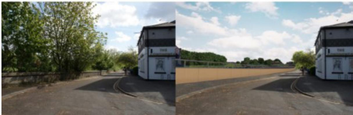
**Preston - Riverside:** Replacement of the existing concrete wall (left), with a new concrete wall with glass panels on top (right), running on the river side of the road in front of the Continental Public House restaurant.
