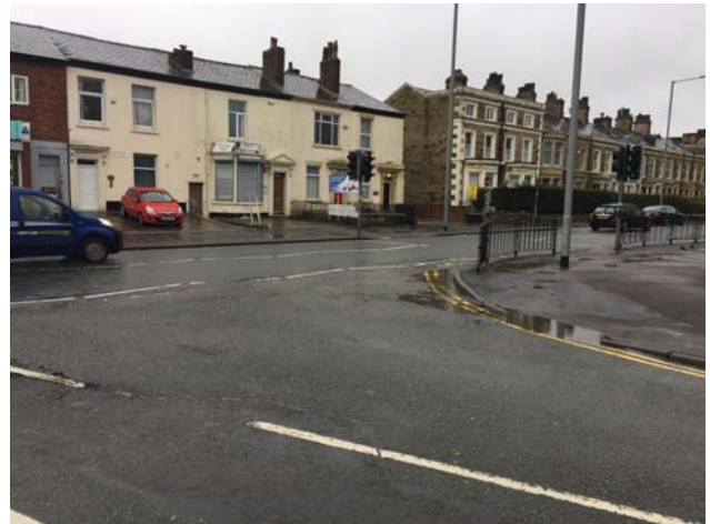
Meadow St / Deepdale Road junction – Pedestrian crossing facilities are in place but there is no provision for crossing Deepdale Road by cycle. Junction redesign is recommended to accommodate both pedestrian / cycle crossing to allow a coherent route from Meadow Street to Peel Hall Street.
