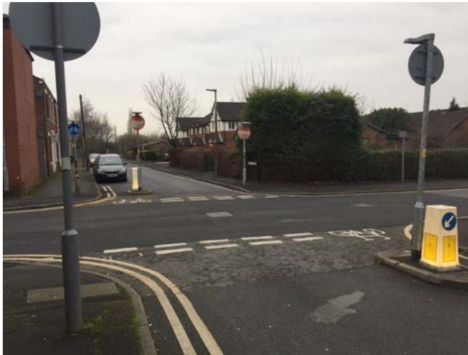
Priory Street / Ashton Street junction – the 'No Entry' except cycles bypass is narrow with vehicles parking in close proximity making it difficult to negotiate, especially for non-standard cycles. Minor works to widen the bypass should be undertaken. Also investigate potential for switching the give-way priority to Ashton Street.
