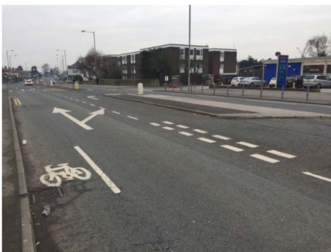
Blackpool Road at Lea Road Junction approach – wide carriageway with substandard width on road advisory lanes. Proposals would reallocate road space for dedicated segregated cycle lanes and incorporate pedestrian crossing facilities at junction, improving access to local supermarket.
