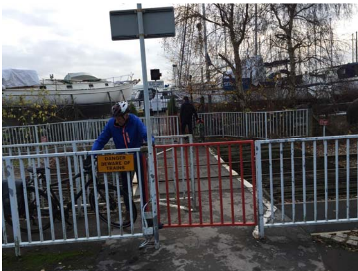
Level crossing – Current arrangement is very difficult to negotiate particularly if using an adapted bike / mobility scooter. Trains appear to run very infrequently and facility should be redesigned to prioritise pedestrians / cyclists outside of times of rail operation.
