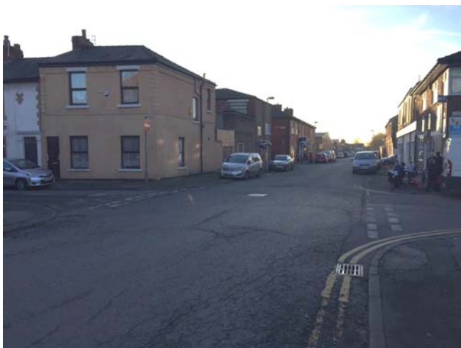
Inkerman Street / Eldon Street Junction – Wide junction requires treatment to reduce crossing distances and simplify for pedestrians / cyclists, incorporating formalised crossing points.
