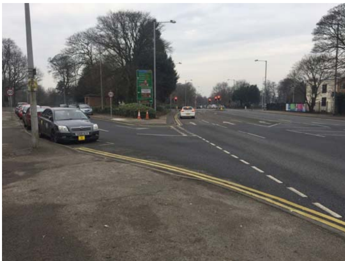
Blackpool Road / Parkside junction – Wide junction mouth to be narrowed reducing turning vehicle speeds and providing increased space for pedestrians. Potential for side road priority treatment
