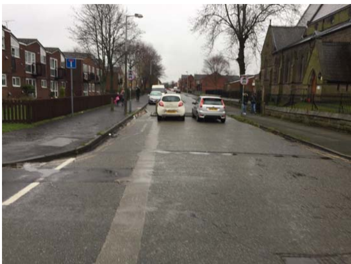
Fletcher Road – Filtered permeability is in place although there is insufficient space for adapted non-standard cycles to pass. Minor works here should be undertaken to increase the available passing space.
