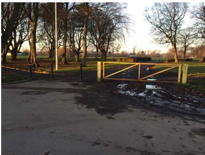
Moor Park Avenue – Area requires maintenance to reduce puddling and remove detritus. Gate could be replaced with access bollard to improve public realm. Wayfinding improvements also recommended as junction of Route 3 and Route 4
