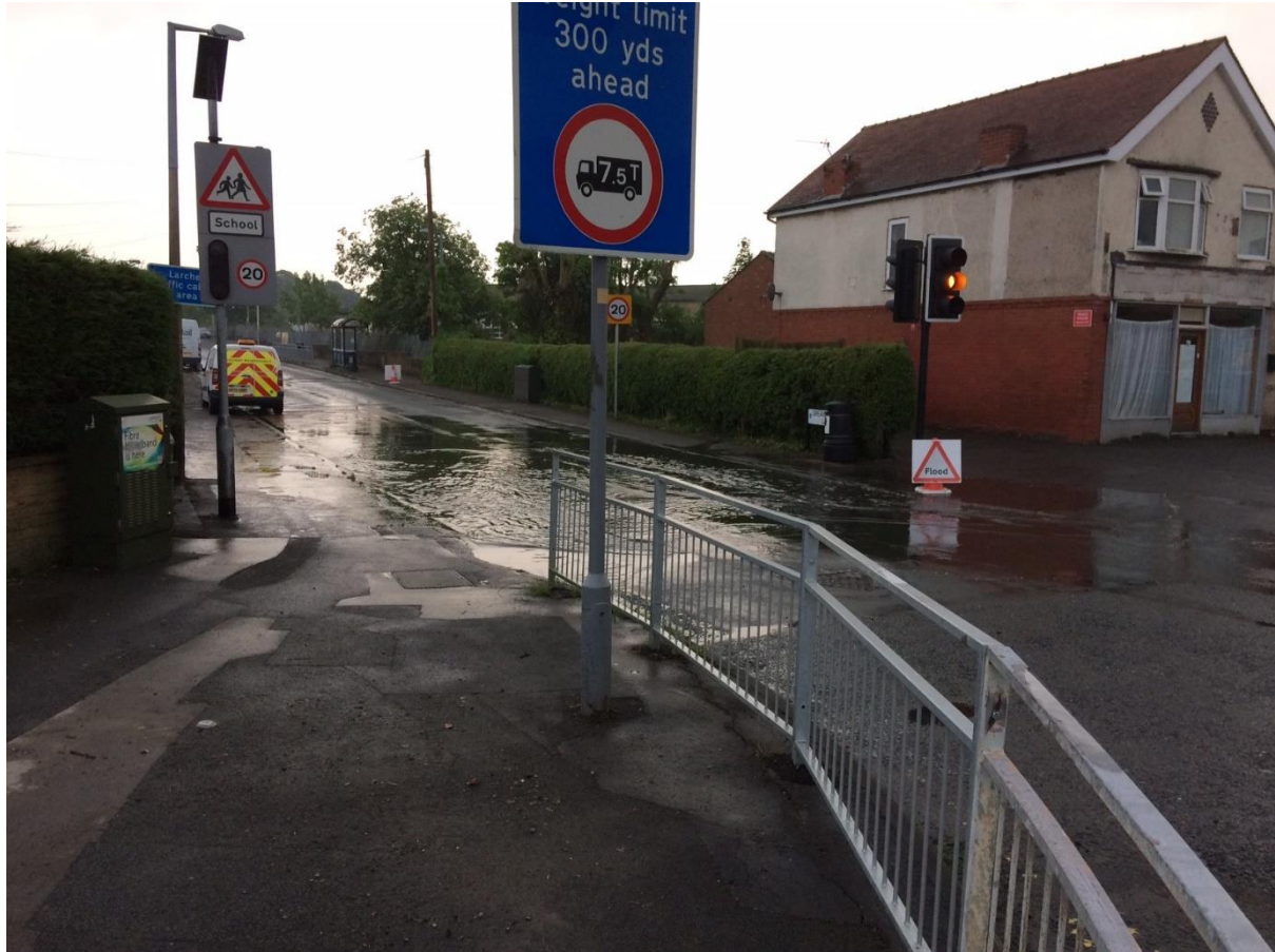
Fig.2 – Emergency response to report of flooded road, Greaves Town, Preston
