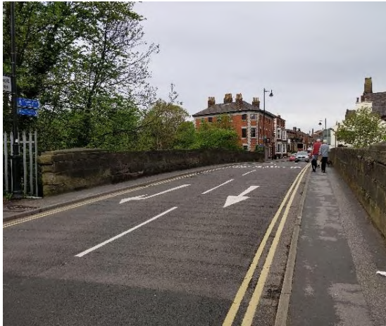
A570 Derby Street bridge
