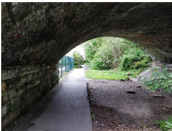
Section of the path, close to the rail station, beneath Derby Street road bridge
