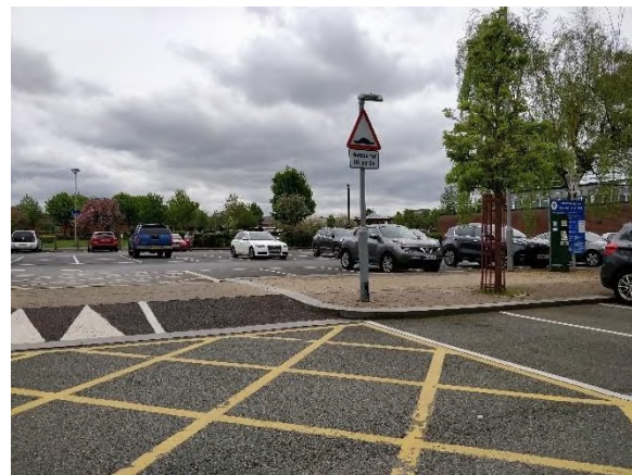
Park Pool car park
