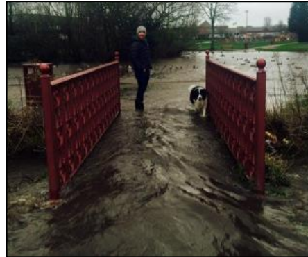
Surcharged brook inundating a footbridge within the park
