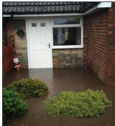
Flooding at a property on Asmall Lane
