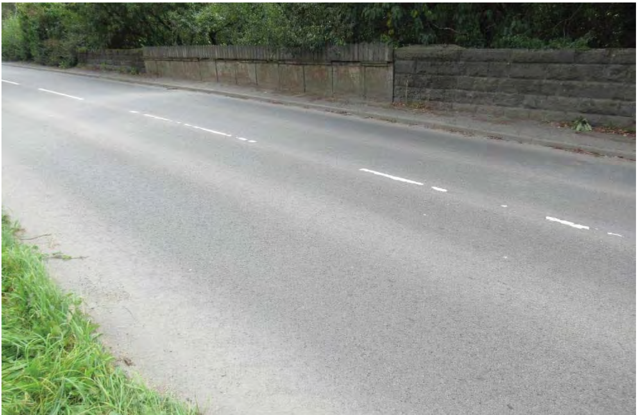
4. Road over deck
