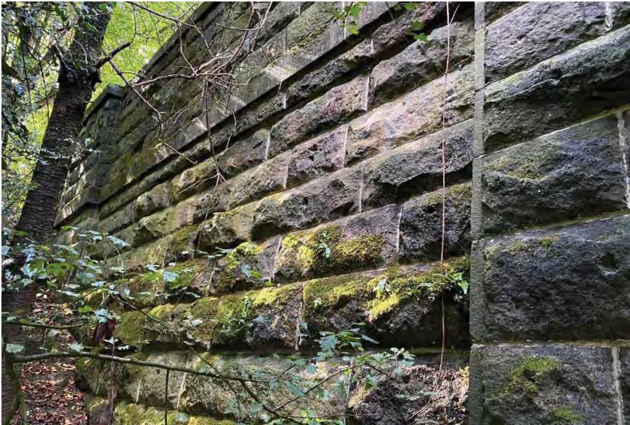
10. South east wingwall
