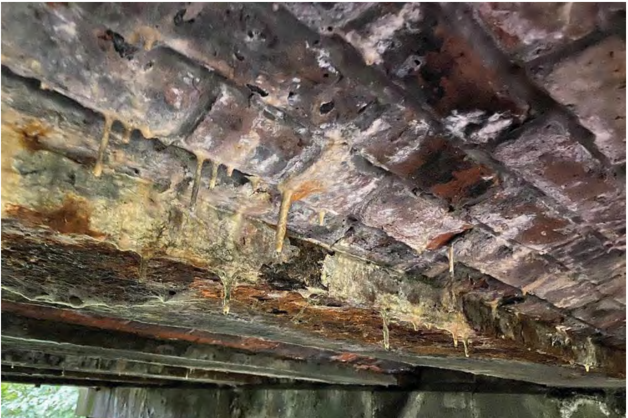
16. Calcite deposits and stalactite formations on jack arches
