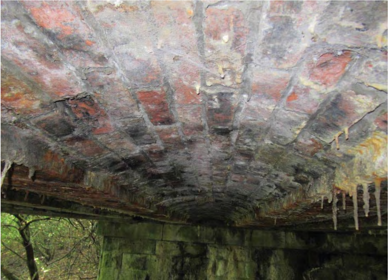
17. Jack arch profile distortion
