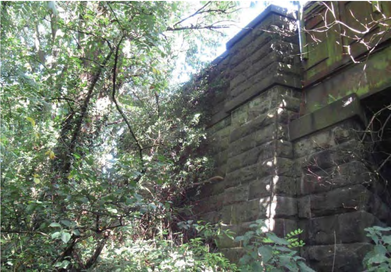
11. North west wingwall
