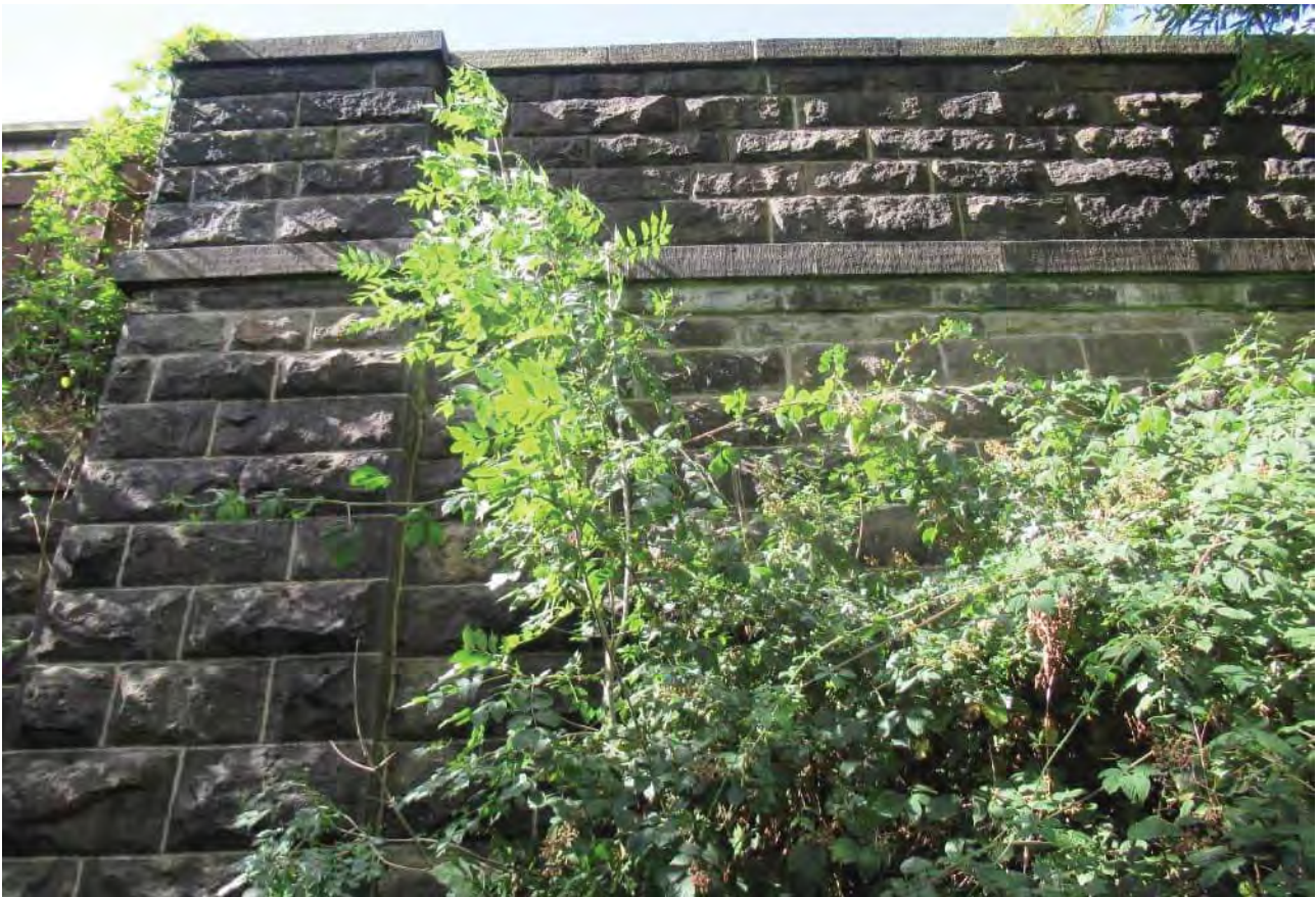
9. North east wingwall
