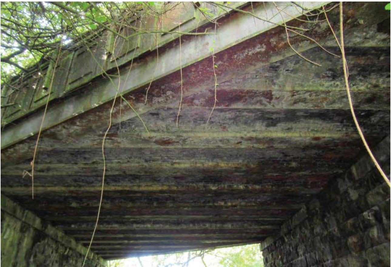
6. General soffit view
