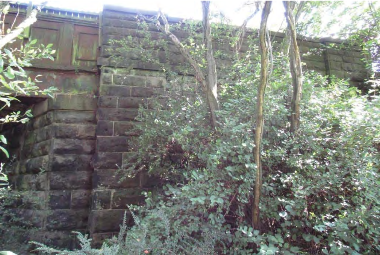
12. South west wingwall
