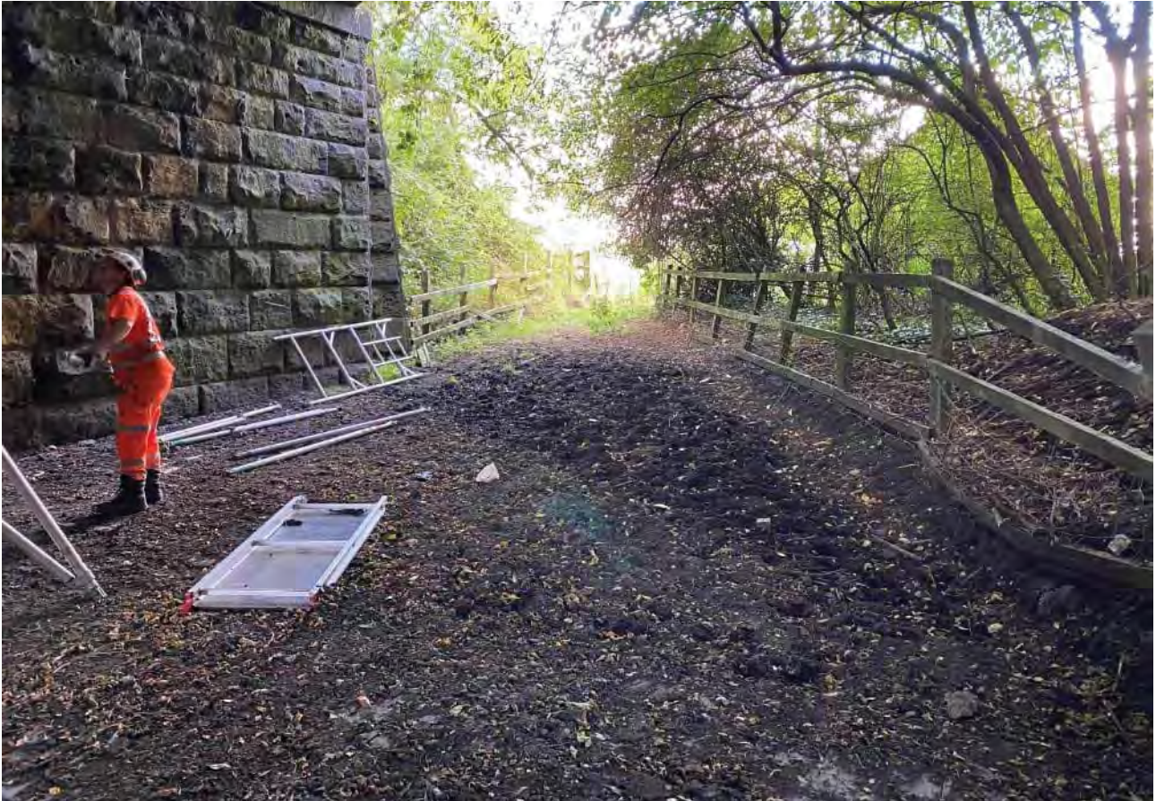
27. View along formation looking east
