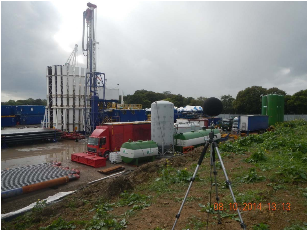
Photograph C1-1: Noise logger on the perimeter bund, NE corner of site
