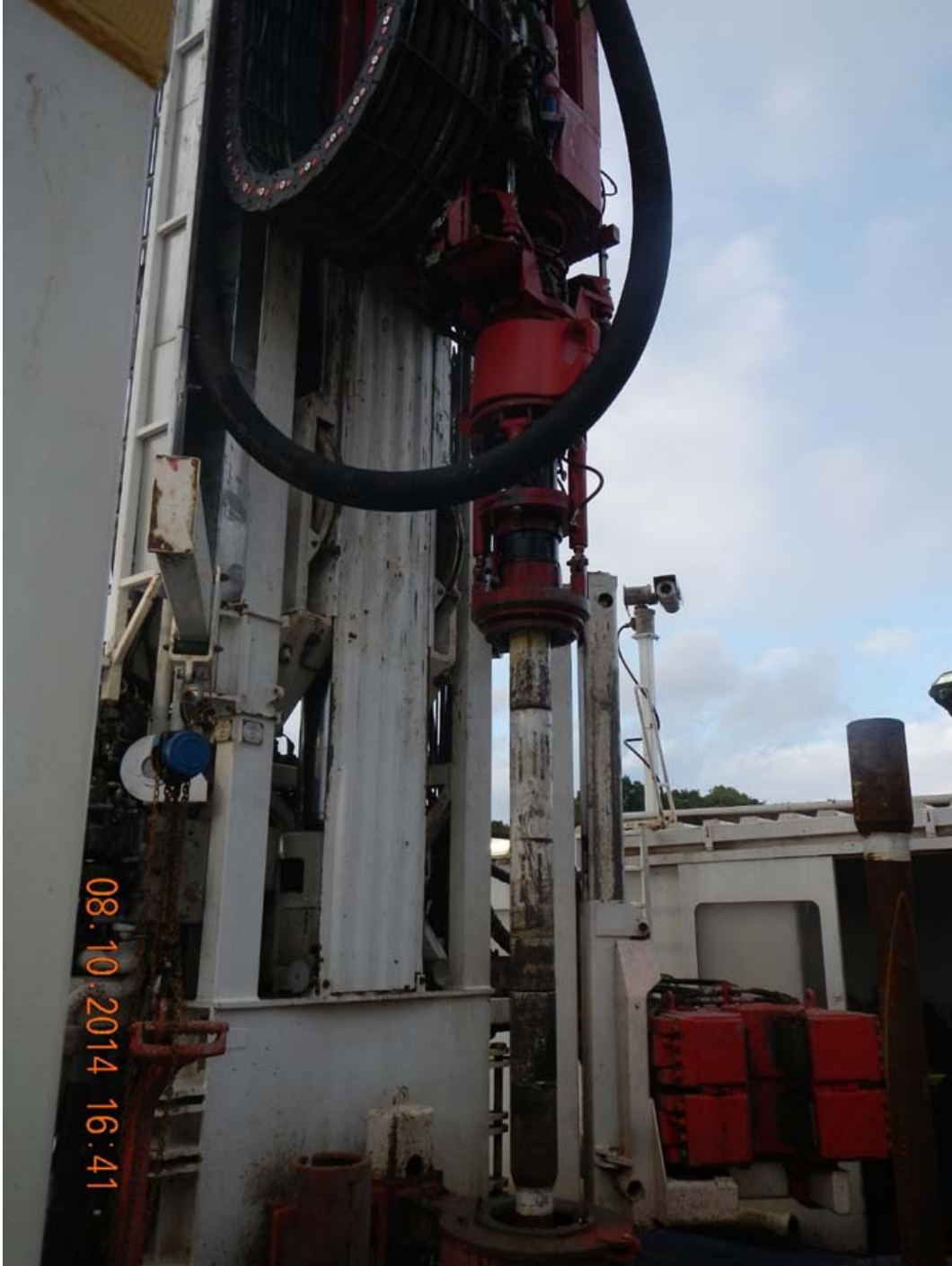
Location 19: Outside Doghouse, approx. 2m from drill string
